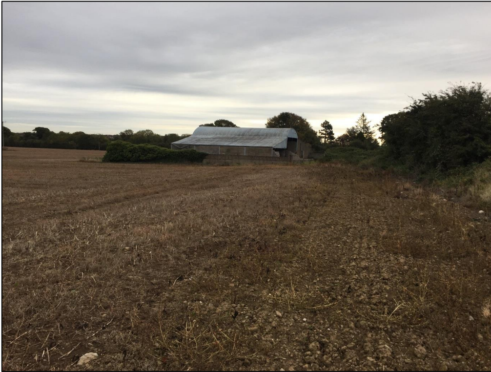
Plate 2: Shed in southern part of subject lands which contains a small roost of common pipistrelle bats.
